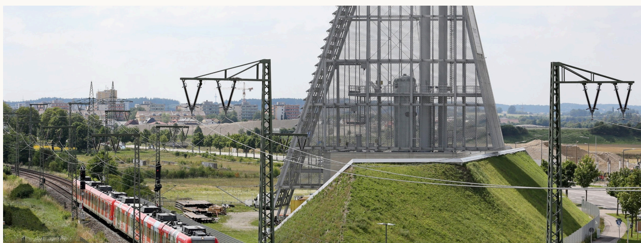
Freiham energy centre, Munich: district-scale climate-neutral infrastructure illustrates the compact, locally led, low-carbon model, set against the market-driven model accelerating elsewhere. Photograph: Landeshauptstadt München / Nagy.
